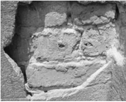
Fig. 5. Randolph Hall, area of bricks and mortar behind stucco that was exposed as part of testing. Samples of both mortar and stucco were removed from this location for laboratory analysis. Photograph by D. Krotzer.
