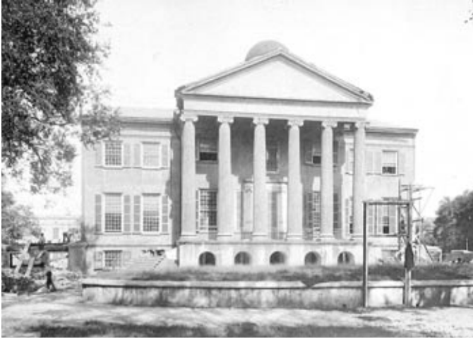
Fig. 3. Randolph Hall in 1887, following the Charleston earthquake. Note that the wings built in 1851 had to be completely removed but that the central portion of the building remained relatively unaffected. Photograph from George L. Cook, Earthquake News , No. 129, courtesy of Photographic Archives, South Caroliniana Library, University of South Carolina.
