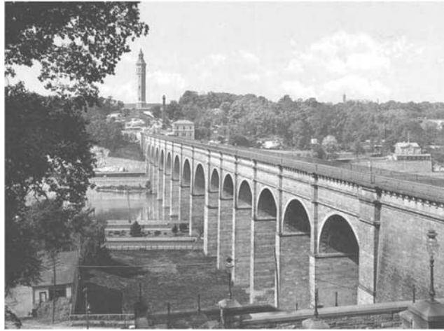
FIG. 1— High Bridge over the Harlem River in New York City. The photograph was taken before 1927 when masonry piers over the river were removed to accommodate a steel span to allow for larger naval ships to pass. The picturesque New York landmark was constructed using Rosendale cement manufactured several tens of miles north along the Hudson River.
